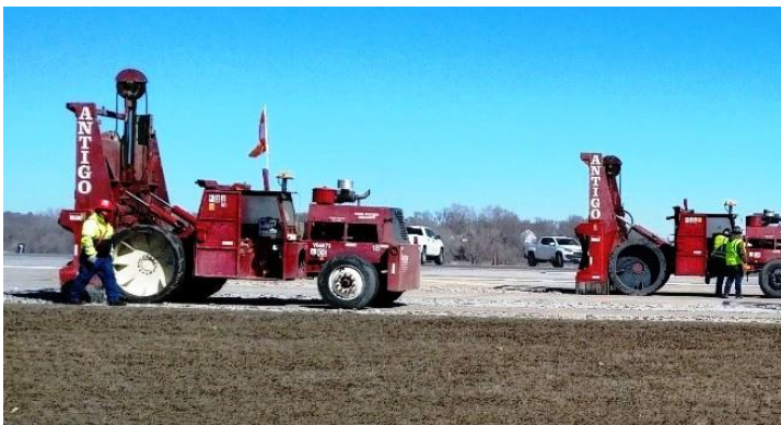
Big 'chines ready to bust up concrete and move dirt.
