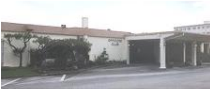
O Club with high rise billeting building seen in the far right background.
